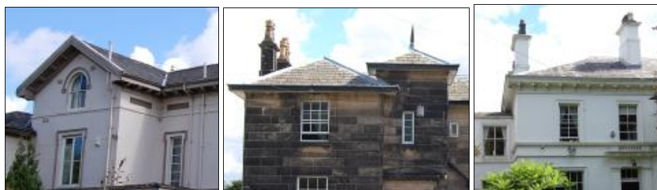
Roof details in the conservation area
