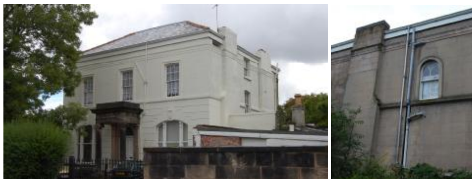
Management issues: (left) a recently painted façade; (right) waste and soil vent pipes, together with a modern fascia treatment.
