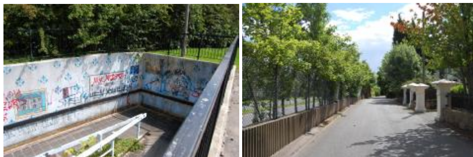
(left) the underpass; (right) wall and fencing alongside the by-pass
