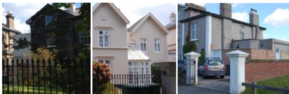
Extensions within the conservation area. The first two images show extensions of a similar form to elements of the original building, but lacking the quality of detailing, the third shows very poor quality and highly visible single storey additions.
